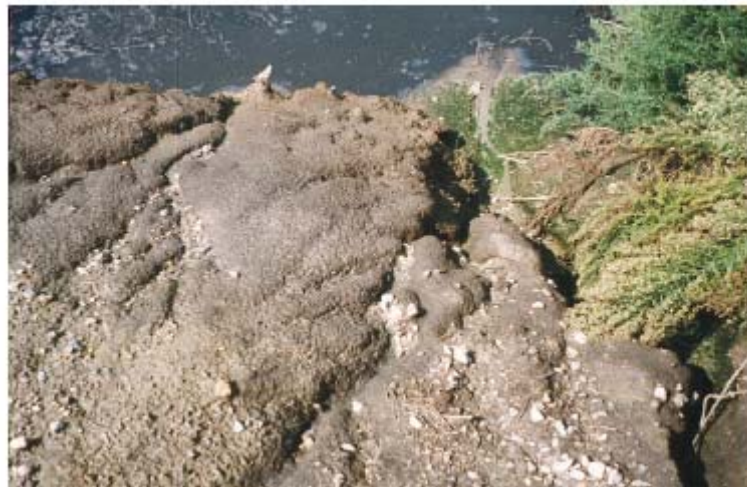
Figure 7-3 Erosion on the inner embankment face of an ELS caused by careless filling of store
