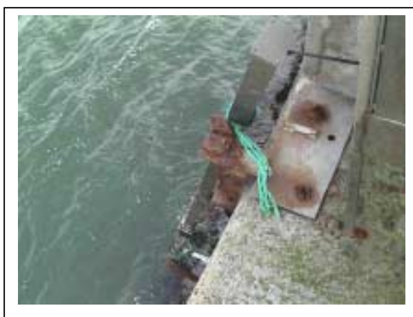
Plate 2.10 Conduit to Pressure Sensor
