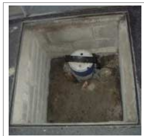
Plate 2.44 Acoustic Sensor
