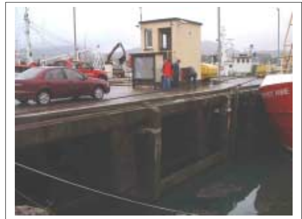
Plate 6.25 Jetty Structure and Control Cabin
