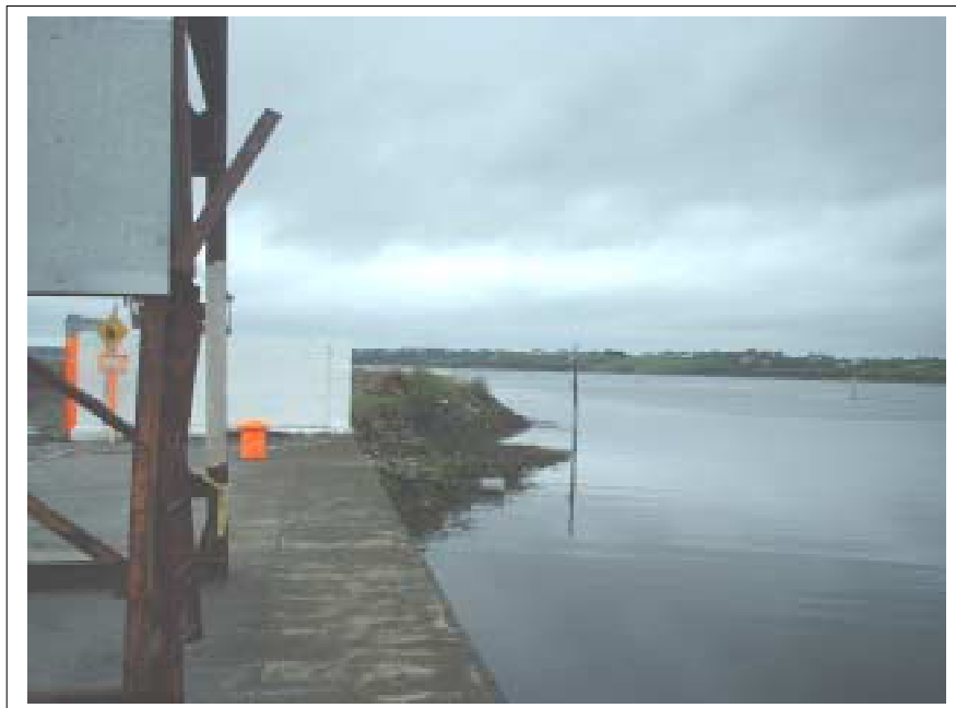
Figure 2.2(c) View from end of quay
