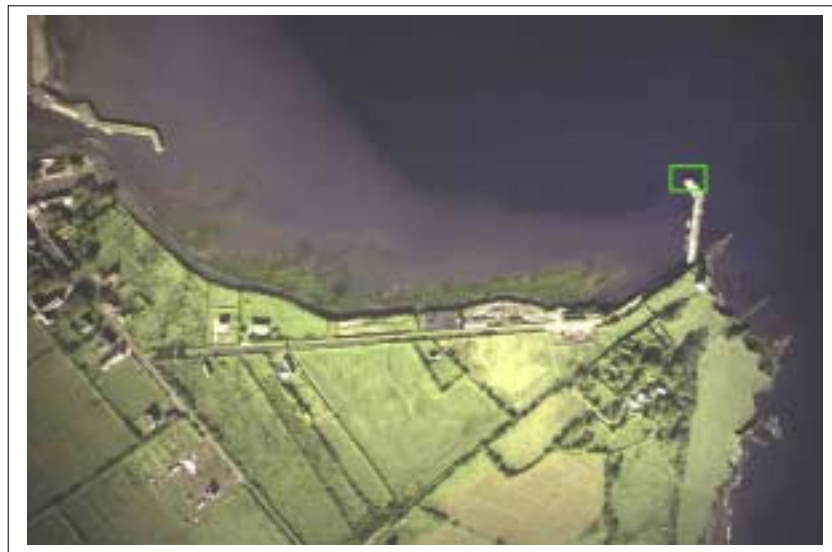
Plate 2.7 Carrigaholt pier showing Gauge location
