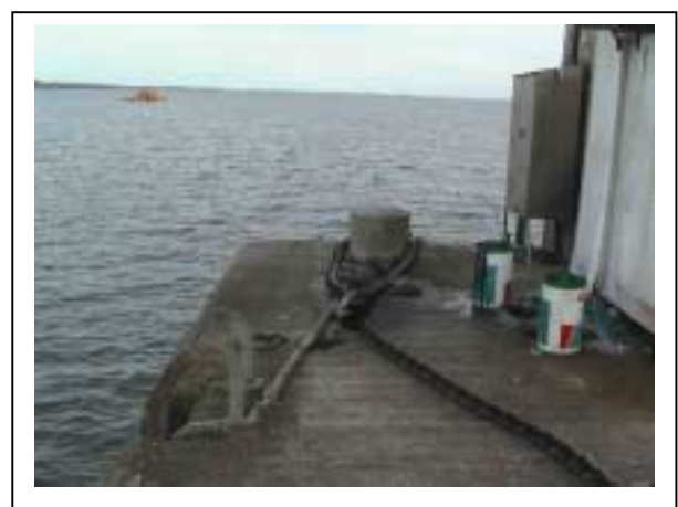
Plate 2.11 Gauge Control Box
