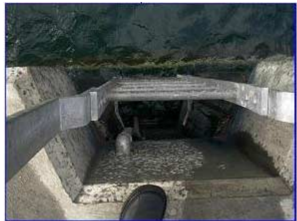
Plate 6.6 Temperature gauge pipe
