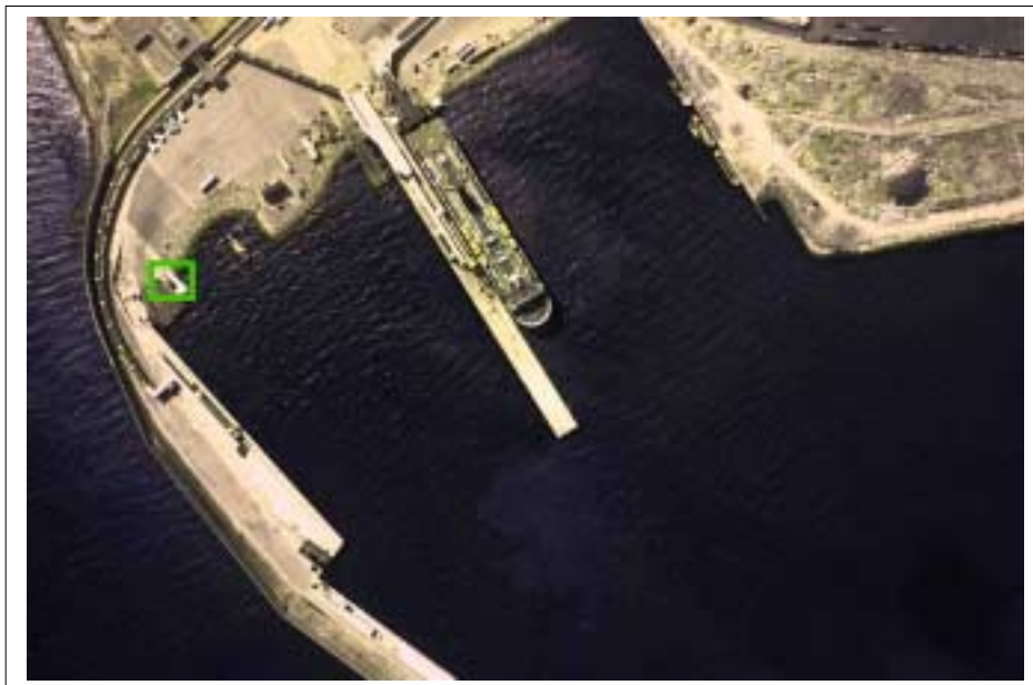
Plate 2.36 Rosslare Gauge Location
