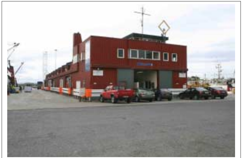
Plate 2.1(b) Killybegs Harbour Building
