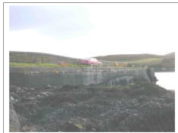
Plate 6.15 Mill Cove Pier – Low tide
