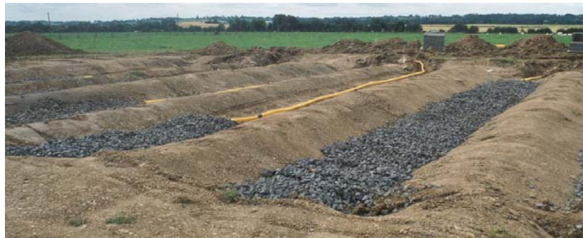
Figure 1: Compacted subsoil ridges in a subsoil-lined OWP effluent collection system
